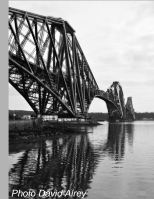
The Forth rail bridge
